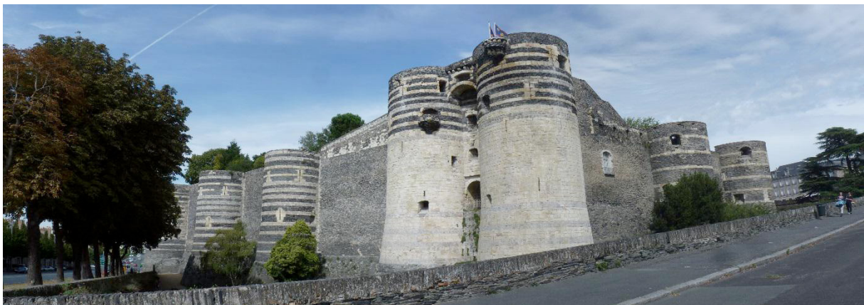
The castle of Angers, black rocks are from the "Anjou Noir" and the white ones from the "Anjou Blanc". Photo: F. Redois.
